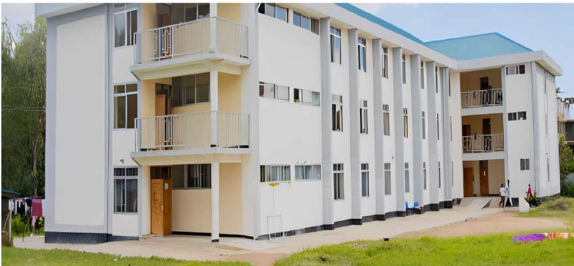
Lake Zone Campus Hostel
